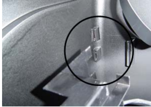
Figure 3.15B LED Assembly groove mount.
